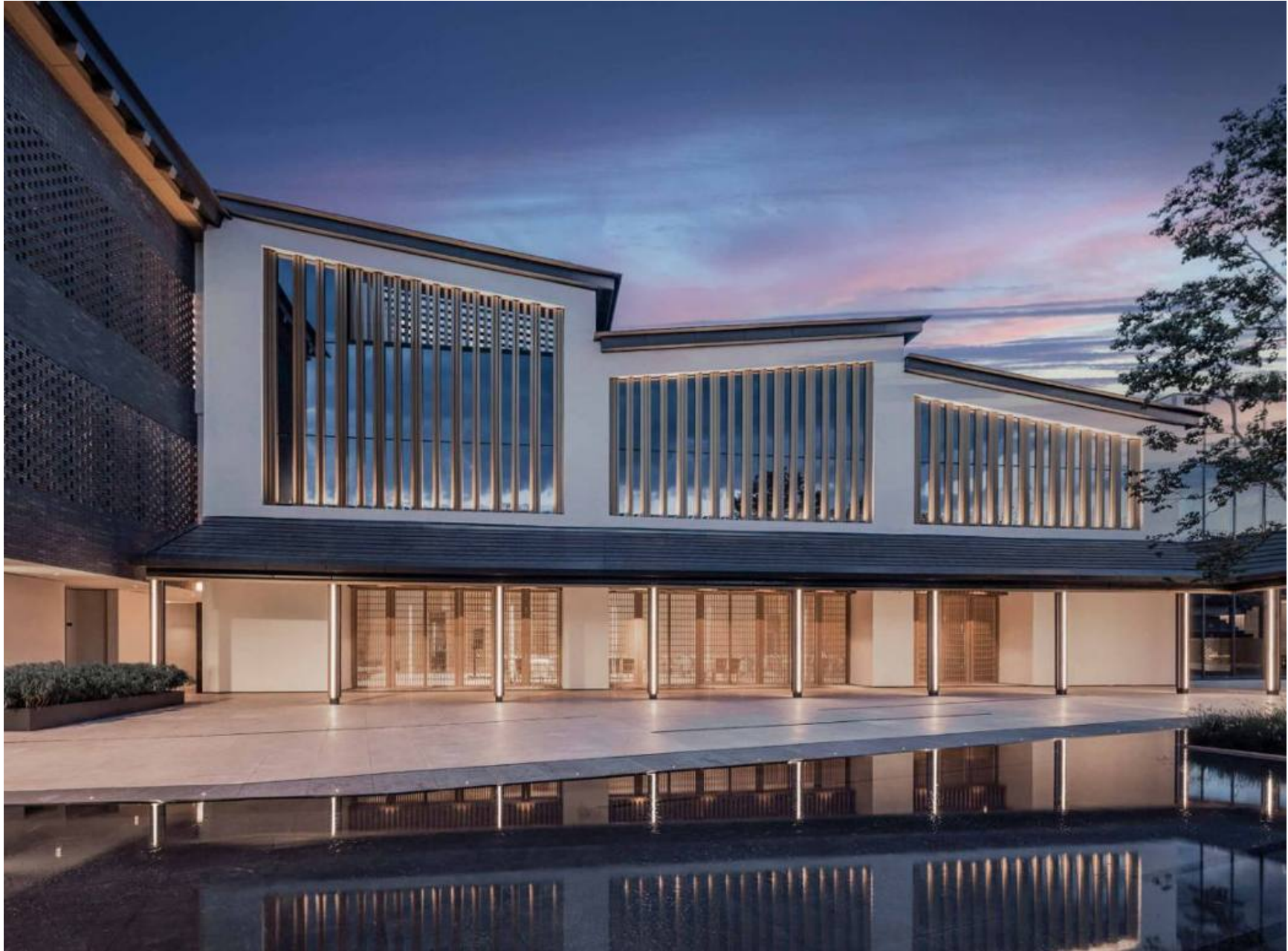
XICHANG VANKE GENERAL CLUB RESORT HOTEL · 外立面黄昏 Facade at Dusk
